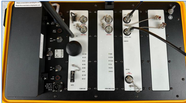
S21 Gain/Loss Setup with connections to Port 1 & Port 2
